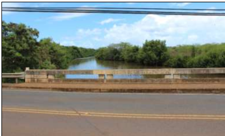
Most bridge stormwater runoff discharges directly to the water bodies below, as seen at this bridge over Ki'iki'i Stream near Waialua
