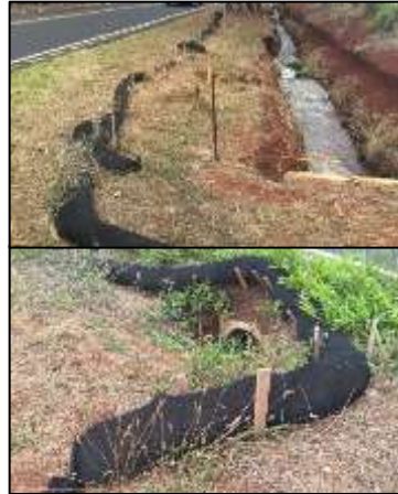
These barriers ("bio-socks") are a temporary BMP placed along Kaukonahua Road help prevent the transport of sediments and other pollutants that are common in runoff from roadways
