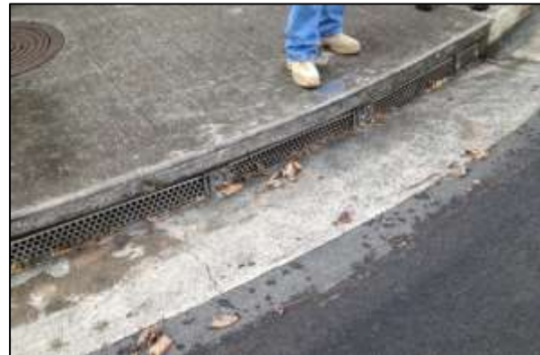
The City MS4 in Wahiawā has filters at some of the stormwater inlets to prevent debris and other pollutants from entering the system
