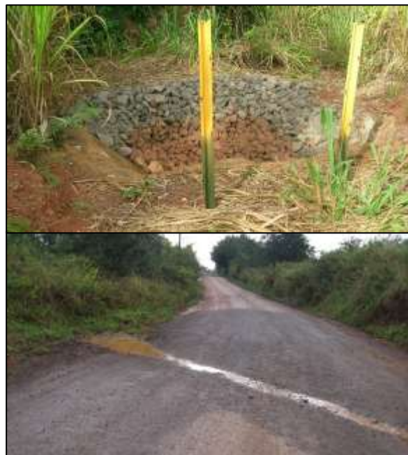
Two examples of practices implemented in Schofield Barracks East Range: Sediment pit (top); Broad-based dip for channeling and directing stormwater (bottom)
